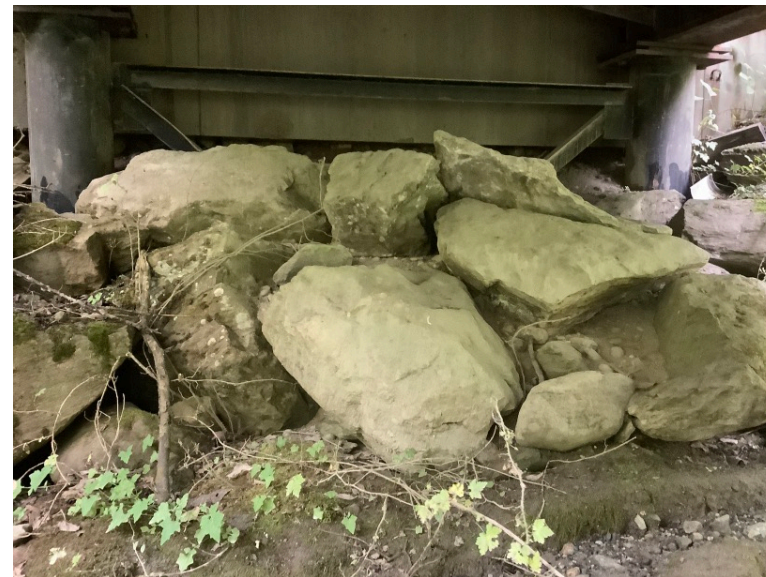
Left Bank Abutment when facing downstream
