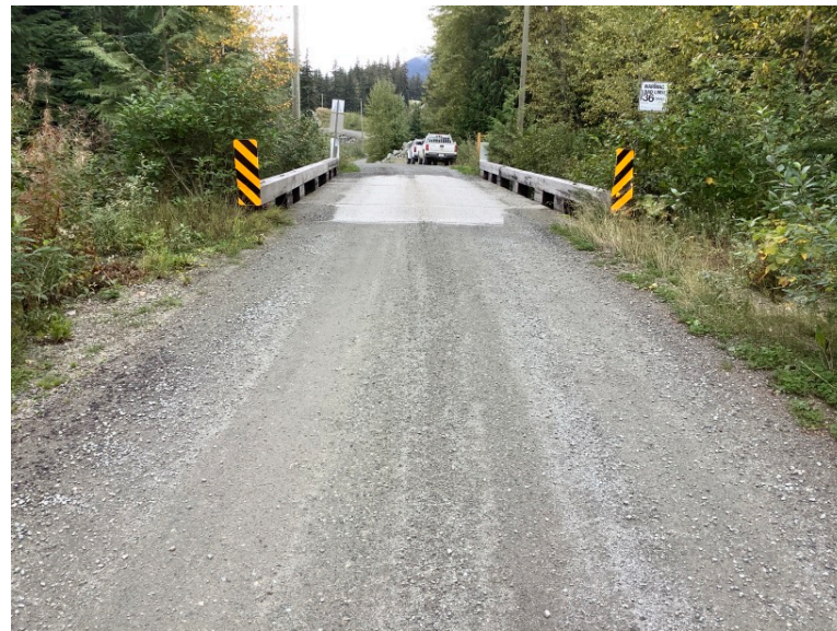
Approach from Left Bank when facing downstream
