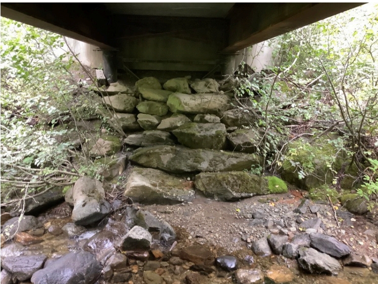
Right Bank Abutment when facing downstream
